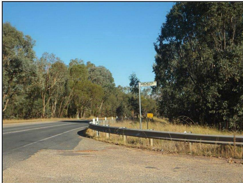
Photo 1: Gerogery Road looking south bound from Winchester Lane.
