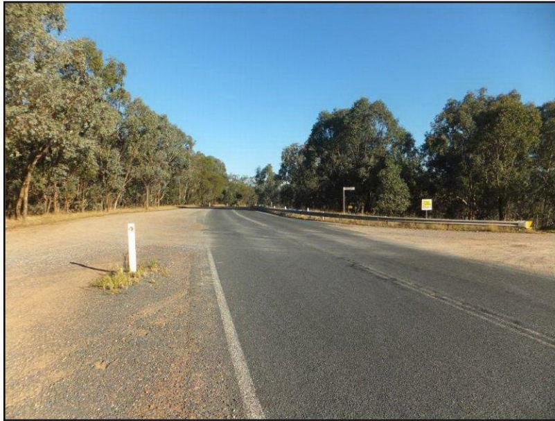
Photo 3: Gerogery Road on top of Nine Mile Hill looking south bound with Winchester Lane access on the right
